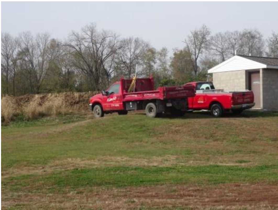
Range 8 Constrution Ongoing And Will Continue As Weather Permits
